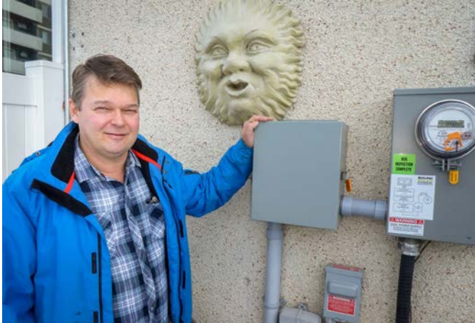
Photo: David Kyle in his backyard with his SaskPower net meter. It monitors both energy consumption and production.
