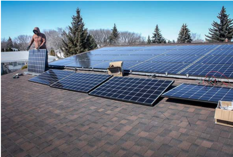
Photo: Installation of solar panels on the roof of David Kyle's home
